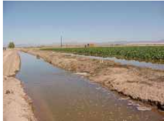
Deep Drain Blocked While Irrigating
