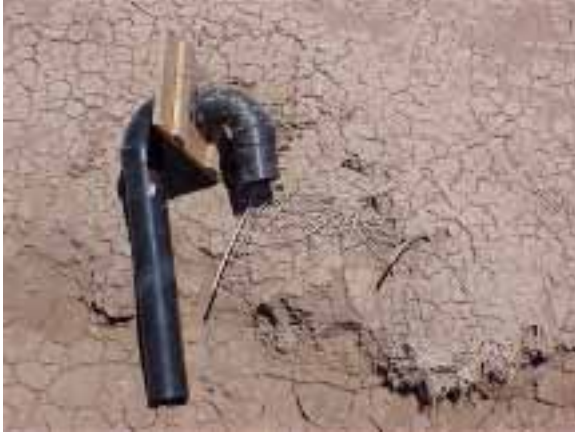
Self-Starting Siphon in Installed In Grade Board
